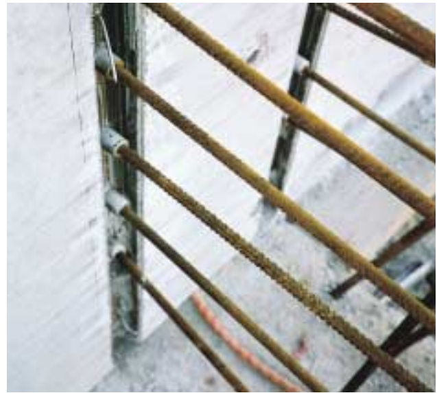
▲ Connections are easy to find after pouring.
