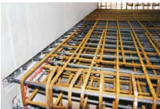
▲ The Coupler box guarantees precise location of the reinforcement bar and additional thrust interlocking.
