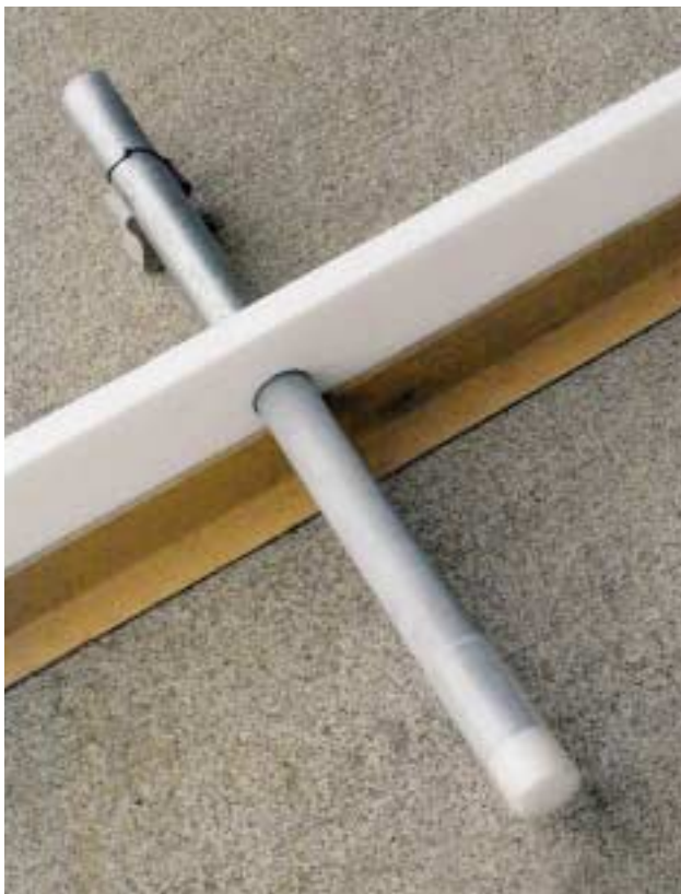
◀ Galvanized dowel, coated one side with expansion space. Fixed in floor slab.
